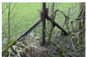
buttressed by other iron struts. Look closely and you will see that they are made out of old broad gauge rails. With the dismantling of the old broad gauge track there were many miles of redundant iron rails
